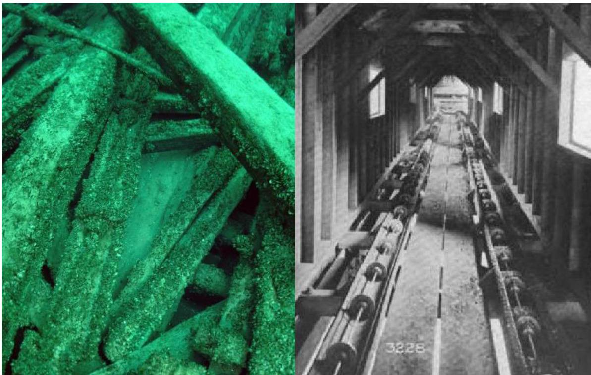
Figure 48. Transfer's cable conveyor (left) and the Jeffery Manufacturing Co. Cable Conveyor (right) (Wisconsin Historical Society; Jeffery Manufacturing Co. 1922)
