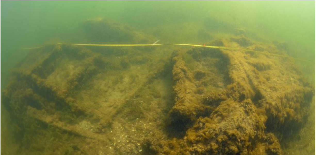
Figure 39. Pan conveyor sections visible above the silt in 2013 (Wisconsin Historical Society)
